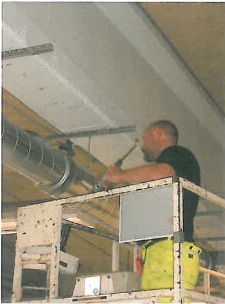
Illustration 7 - Calking the duct system
