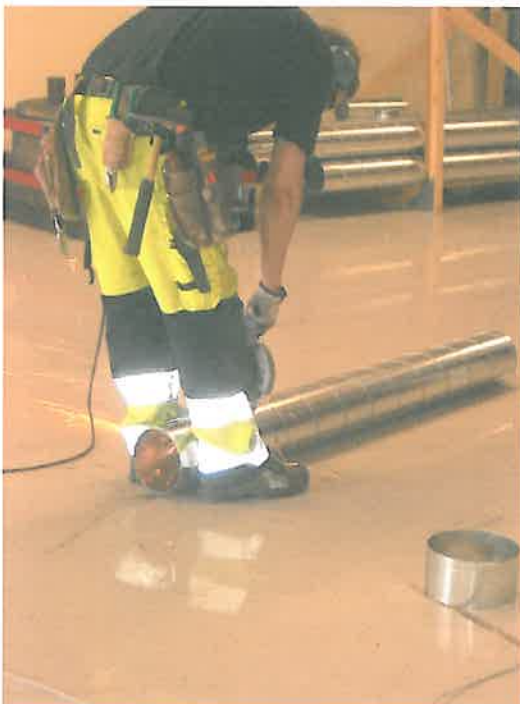
Illustration 1 - Cutting round duct Illustration 2 – Round duct fittings
