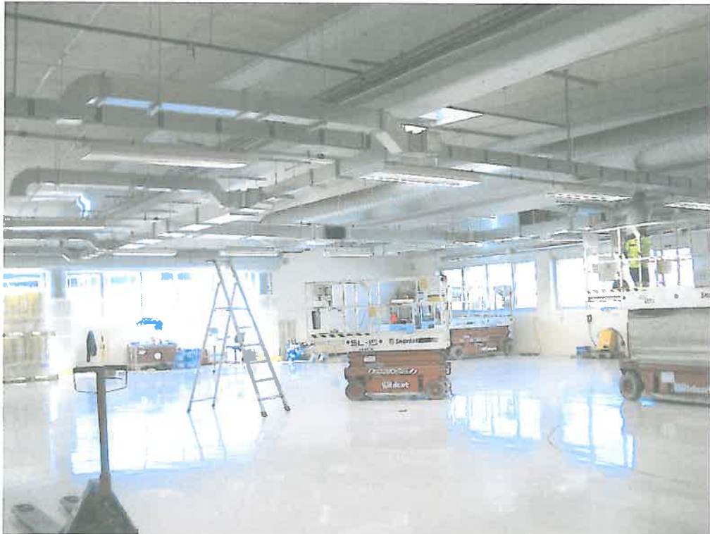
Illustration 19 - Rectangular duct system
