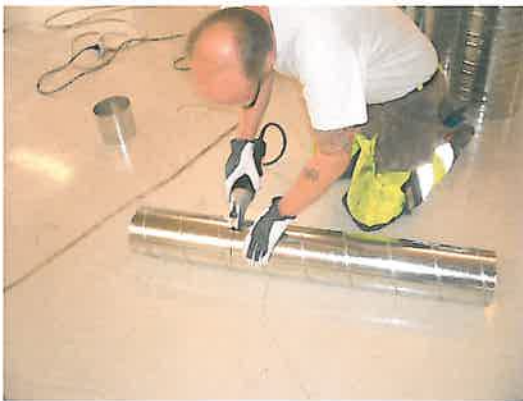
Illustration 6 - Cutting to length
