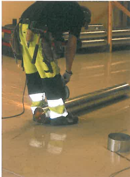
Illustration 12 - Cutting the round spiral duct
