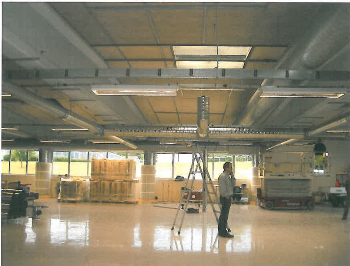
Illustration 16 - Vent with tape/mastic and Safe/Safe-Click systems
