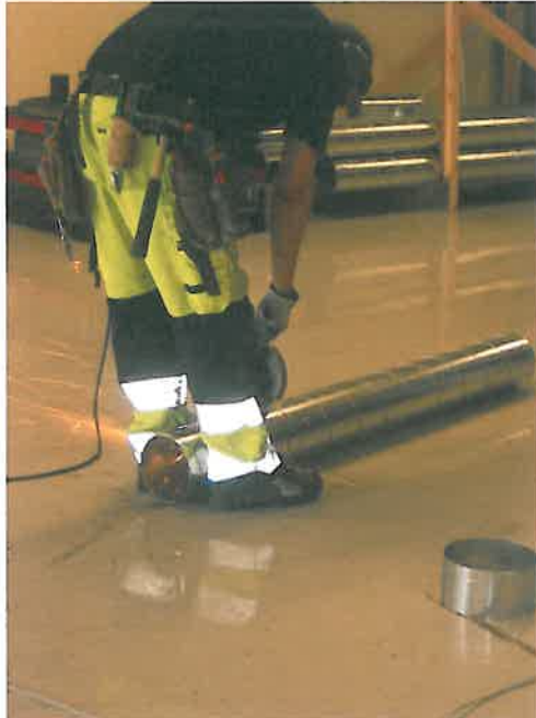
Illustration 5 - Cutting round duct
