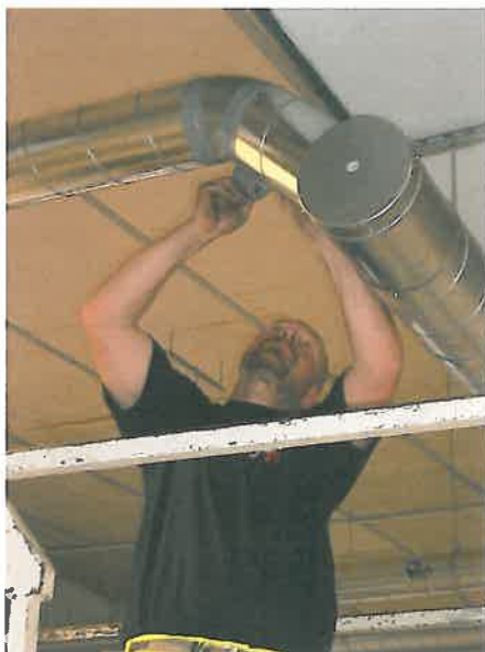
Illustration 3 - Sealing with tape
